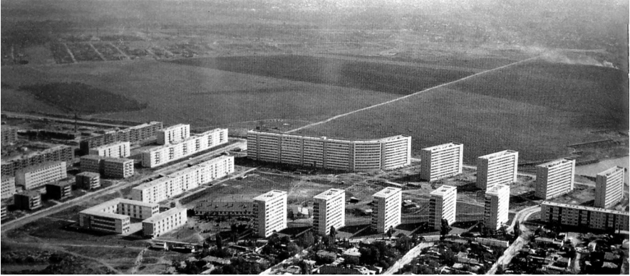
Fig. 6. Aerial view of a microraión in the Balta Albă housing district, Bucharest. Published in Arhitectura RPR 12, no. 4 (1964): 28.
